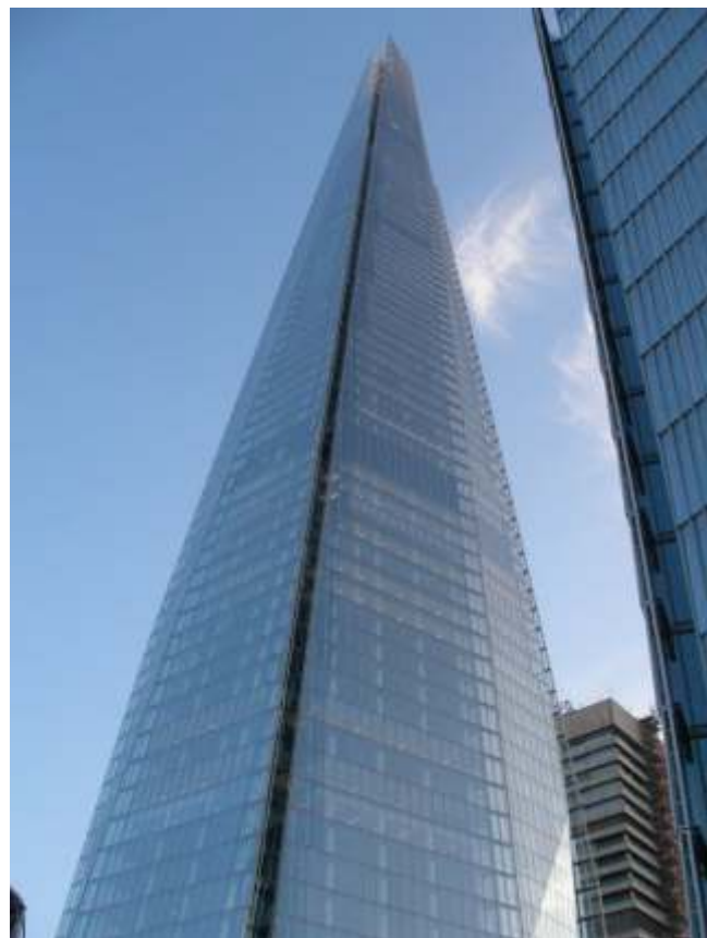
Fig. 2: The Shard is the tallest building in the UK and currently in Europe. The C35/45 concrete contains a cement blend using 70% GGBS to limit early heat generation. This high level of additional cementitious material has the potential disadvantage of low early strength. This was overcome by developing the concrete so that it would achieve sufficient strength to meet initial structural requirements within 14 days with the full strength being achieved at 56 days.
