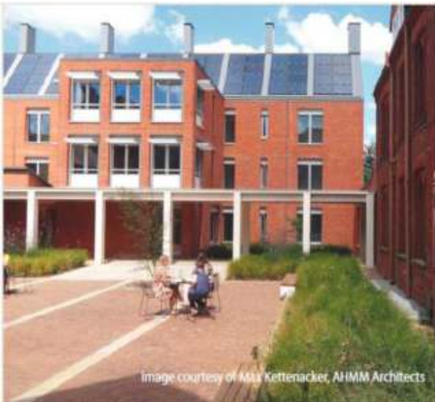
Fig. 4: Ash Court, Girton College, Cambridge. A residential wing providing 50 en-suite bedrooms, gym accommodation and an indoor swimming pool; Resilience to climate change has been addressed by installing plastic pipework in the exposed concrete soffits, allowing active surface cooling to be used in the future. This added little to project costs.
