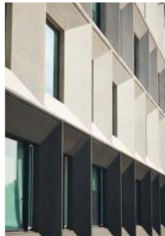
Fig. 3: Burntwood School, London. Precast cladding panels were pre-glazed with insulation added in the factory, significantly reducing wastage; Exposed concrete soffits throughout to provide thermal mass; Concrete slabs, stairs, classrooms, etc. with no finishes provide attractive no-waste no-maintenance hard-wearing surfaces appropriate for a tough school environment.
