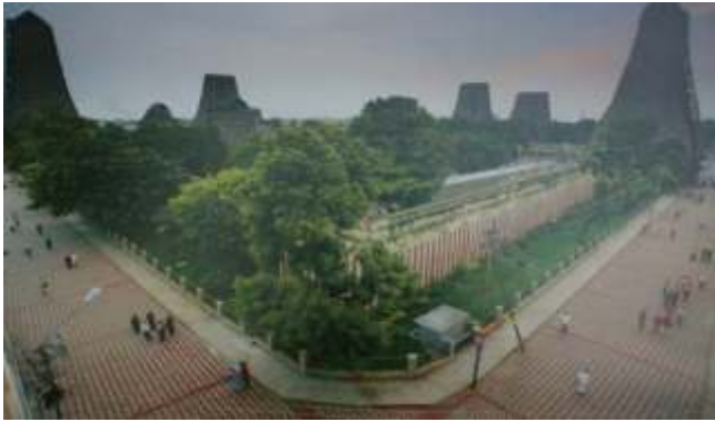
Fig. 9.7: Aerial View of the Existing Pedestrianised Meenakshi Temple surrounds
