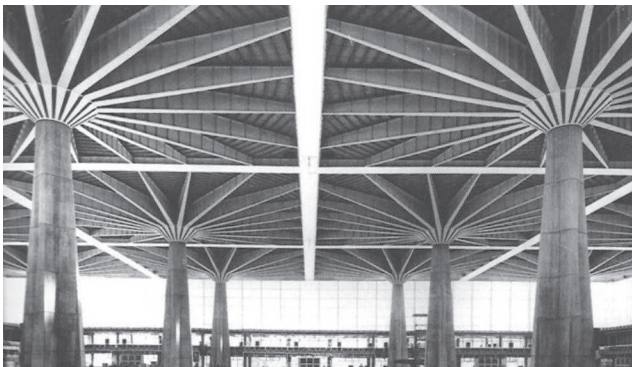
Photo 2: Palazzo del Lavoro in Turin, Italy
