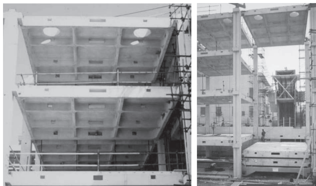
Figure 1 the slabs in the final position Figure 2 lifting of the plate
