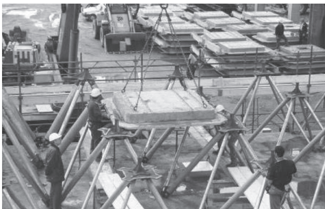
Figure 11 placing of the precast concrete forms over joints
