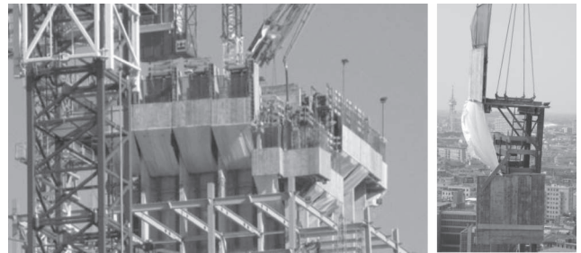
Fig. 4 - Climbing Formwork System
