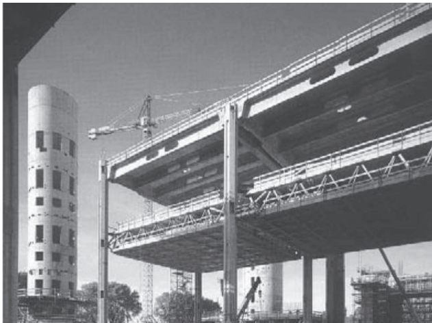
Figure 8 roof units in position over the floors
