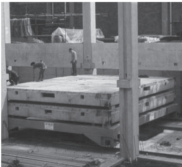
Figure 3 stacking the plates over the launching cart
