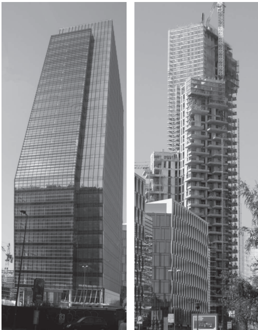
Fig. 3 - Construction Site: Bld 3 (left) and Bld 12 (right)
