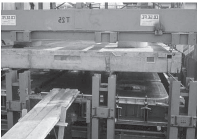
Figure 4 demoulding from the self stressing form
