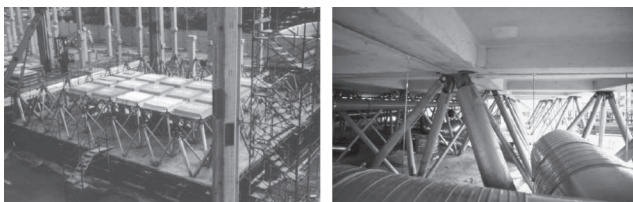
Figure 12 placing of ducts and wirings inside the plate
