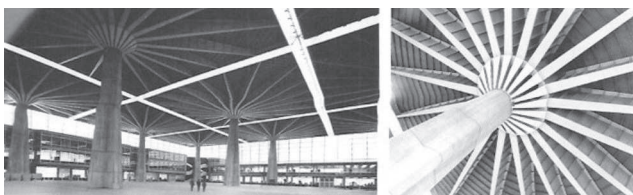
Fig 13: (left and right) Patàzzo del Lavoro in Turin, Italy, 1959-61, Pier Luigi Nervi with Antonio Nervi and Gino Covre
