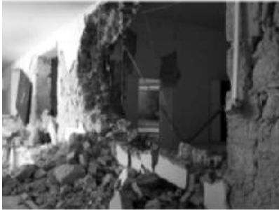
Figure 4: Severe shear cracks and collapses in the internal walls of the South-East wing
