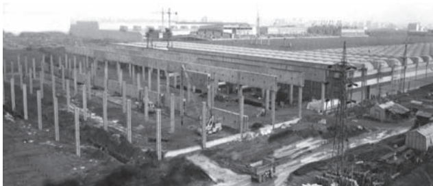
Figure 5. View of the construction of the assembly building
