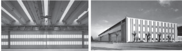
Figure 8. Inner and outer views of the hangar
