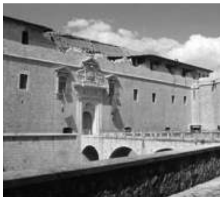
Figure 3: Out-of-plane overturning of the upper part of the main façade (South-East side)
