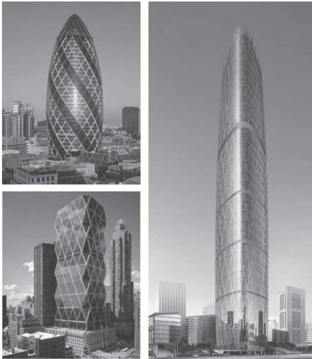
Figure 5. Case studies; top left) Swiss Re; down left) Hearst Tower; right) Guangzhou West Tower
