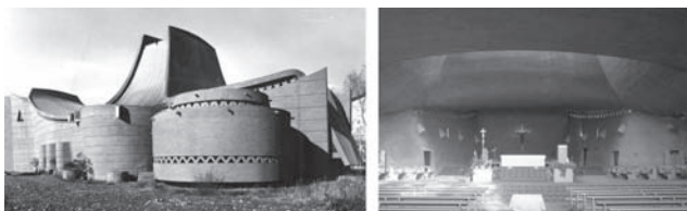
Figure 2. Outside and inside view of the church
