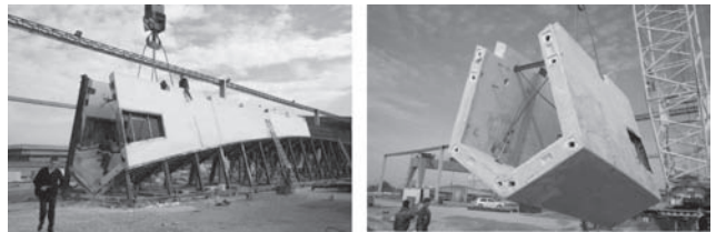
Figure 11. "Matching Concrete" casting technique for the ribs and element being hoisted
