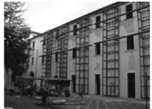
Figure 5: Provisional interventions carried out on SE and SW wings: connection of the internal and external façades by means of steel cables and steel frames against the façades.
