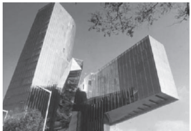
Fig. 5: General view of the complex
