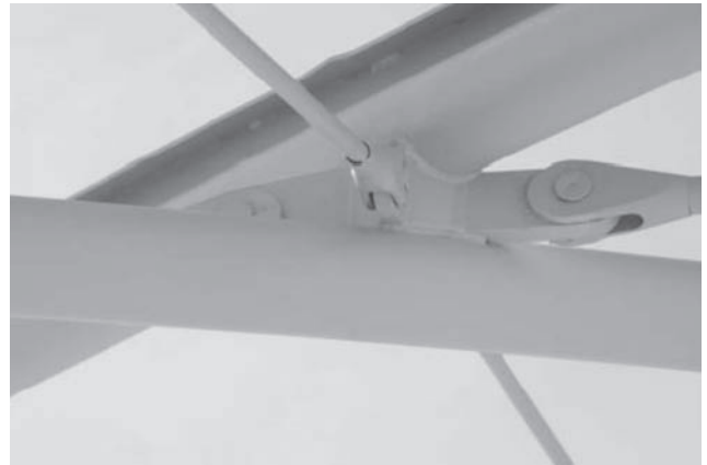
Fig. 15: Detail of the joints between dome layers
