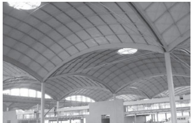
Fig. 17: Inside view of the dome system
