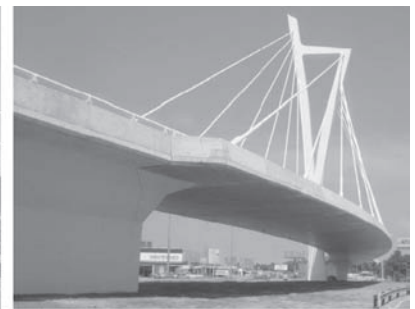
Fig. 29: Continuity of the deck
