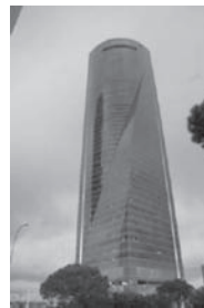
Fig. 10: Tower with open concourse on ground level
