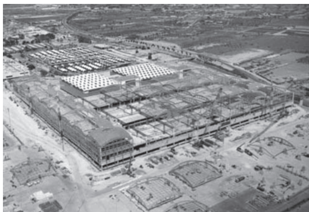
Fig. 14: Bird's eye view of the construction process
