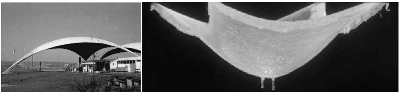
Figure 7: Concrete Shell by Isler and experimental funicular model
