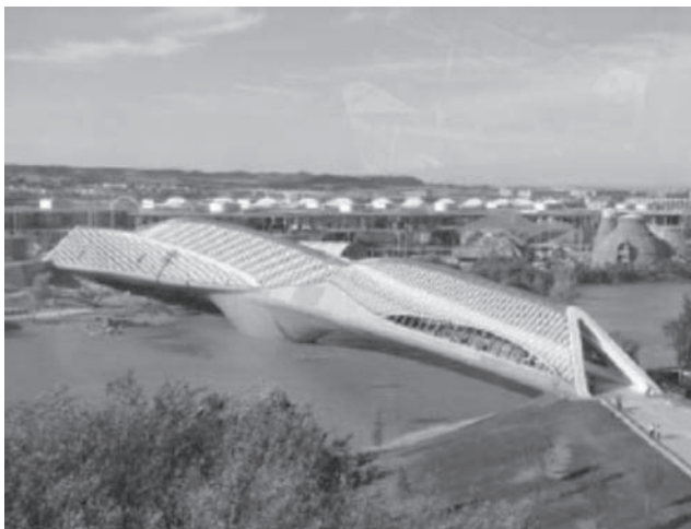
Fig. 2: Zaragoza Pavillion-Bridge (Zaha Hadid); Bird's eye view
