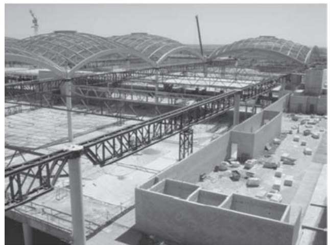
Fig. 16: Placement of domes through launching on provisional girders
