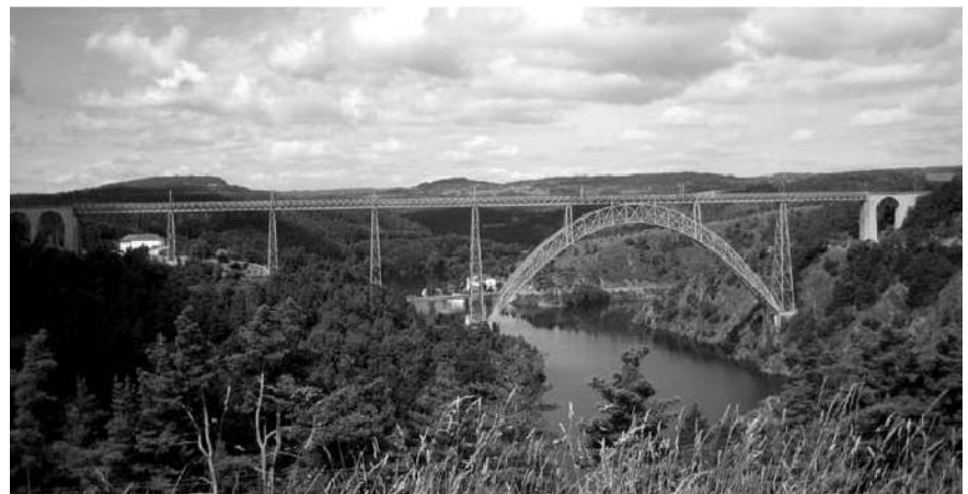
Figure 5 : Garabit Viaduct Gustave Eiffel
