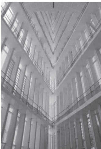
Fig. 26: Inner patio with special horizontal bracing beams
