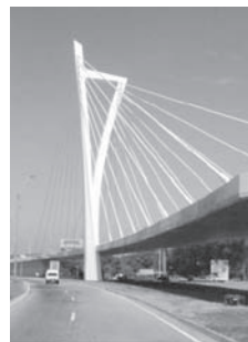
Fig. 28: External view with pylon
