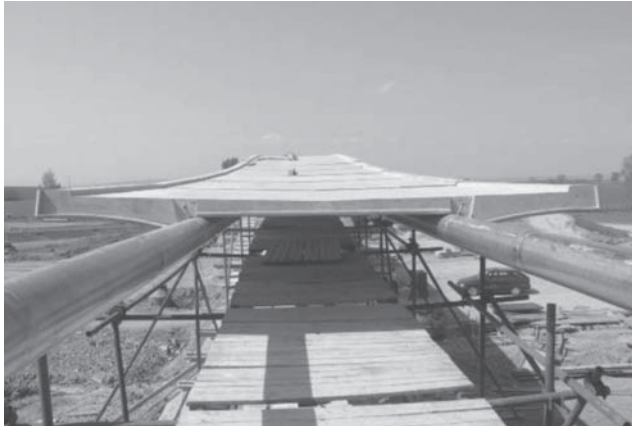
Figure 2: Segments on external cables
