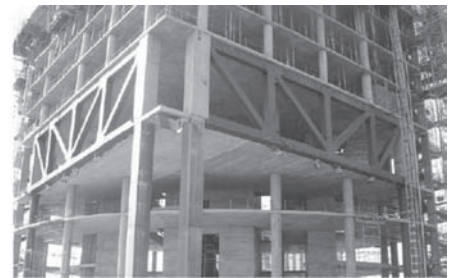
Fig. 11: View of the truss girders in the building
