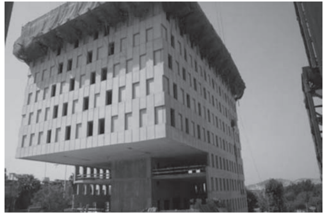
Fig 20: Hotel structure after prop removal
