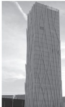
Fig. 25: Arrangement of the double façade members
