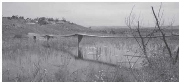
Figure 1: Lake Hodges Pedestrian Bridge
