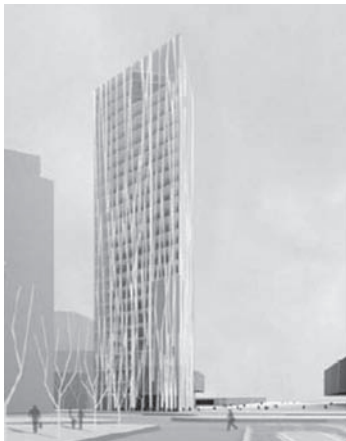
Fig. 24: Model showing the double facade system
